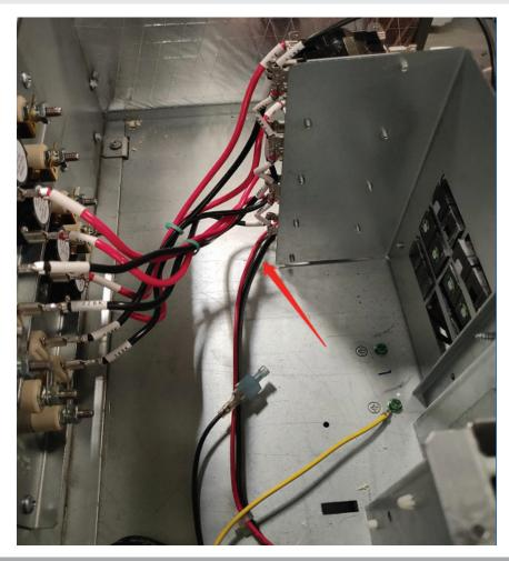
5.) Insert signal wire into the main electronic control board
