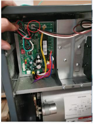
6.) Reinstall the upper side panel. The switches for the heat kit should protrude through the hole you knocked out of the panel. Then, turn on the power and check operation.
