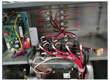
3.) Fasten heat kit electrical board bracket to air handler by installing two screws
