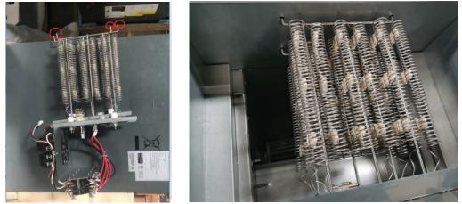
2.) Reinstall screws to fasten the heat kit to air duct
