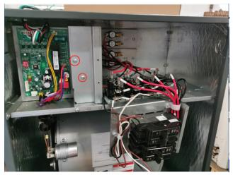
4.) Position the heat kit electrical board on the bracket and fasten with 4 screws
