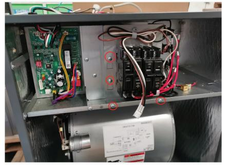
NOTE: When installing the electrical installation board, pay attention to the indoor unit power cord and make sure it does not hang or snag on the sharp edges of the sheet metal heat kit bracket. Please refer to the image below.
