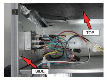
Figure 11. Electrical Connections (Upflow Configuration)
